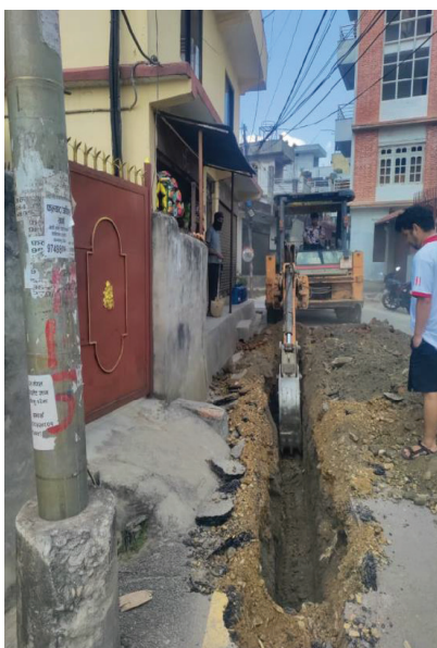
excavation for pipeline
