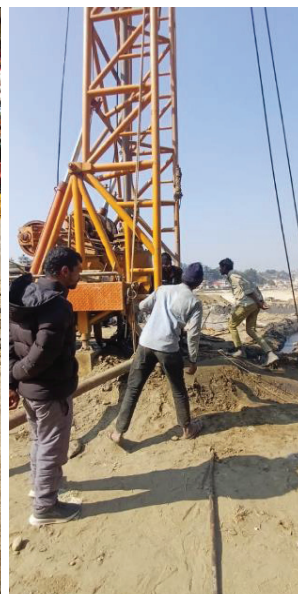
Deep boring works
