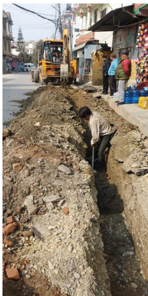
Excavation for pipe laying works
