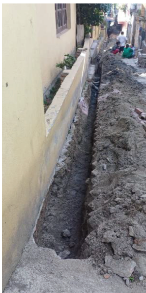
Excavation for pipe laying works
