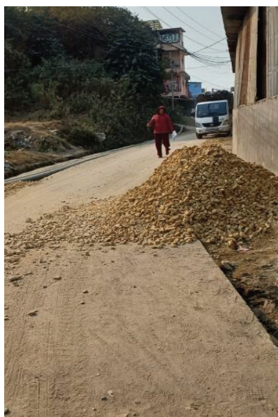
Basework for reinstatement
